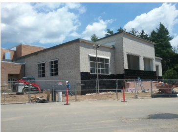
Exterior of CMS STEM Addition
